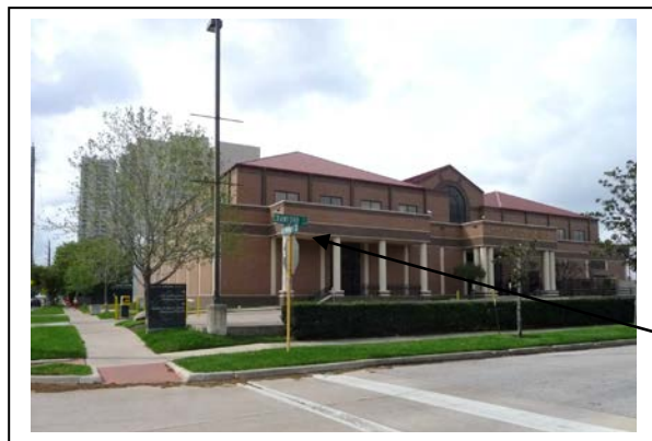
Parking entrance off of Hermann Drive
